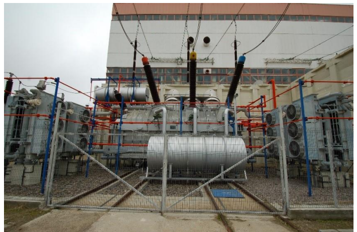
Fig. 17 Transformer 440MVA
