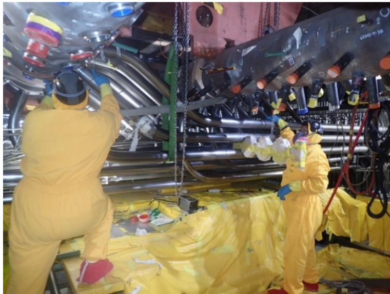
Fig. 11 Installation of upper feeders
