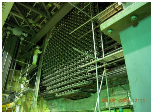
Fig. 8 Dismantling the feeders
