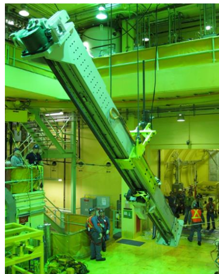
Fig. 9 The platform for dismantling the fuel channels
