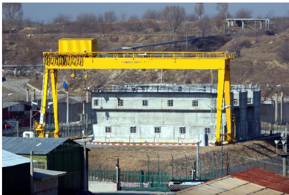
Fig. 6 The intermediate storage of dry spent fuel
